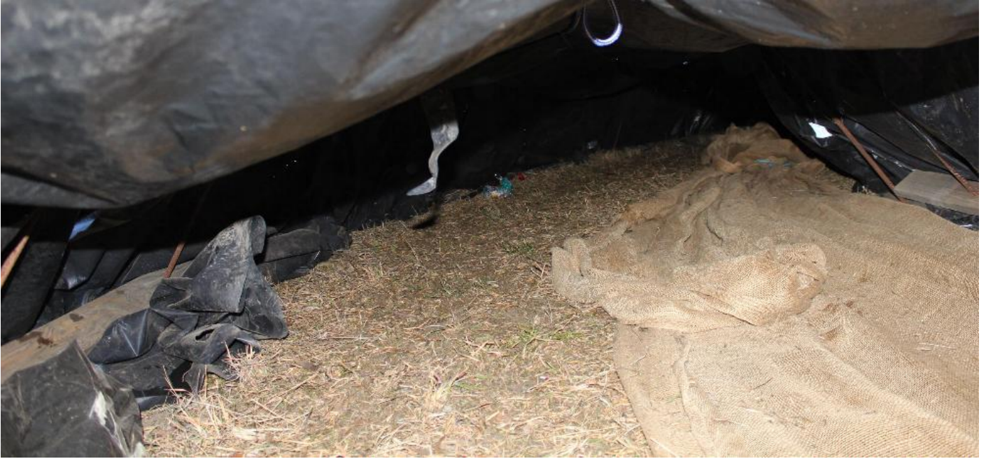
(looking back inside the tunnel)
